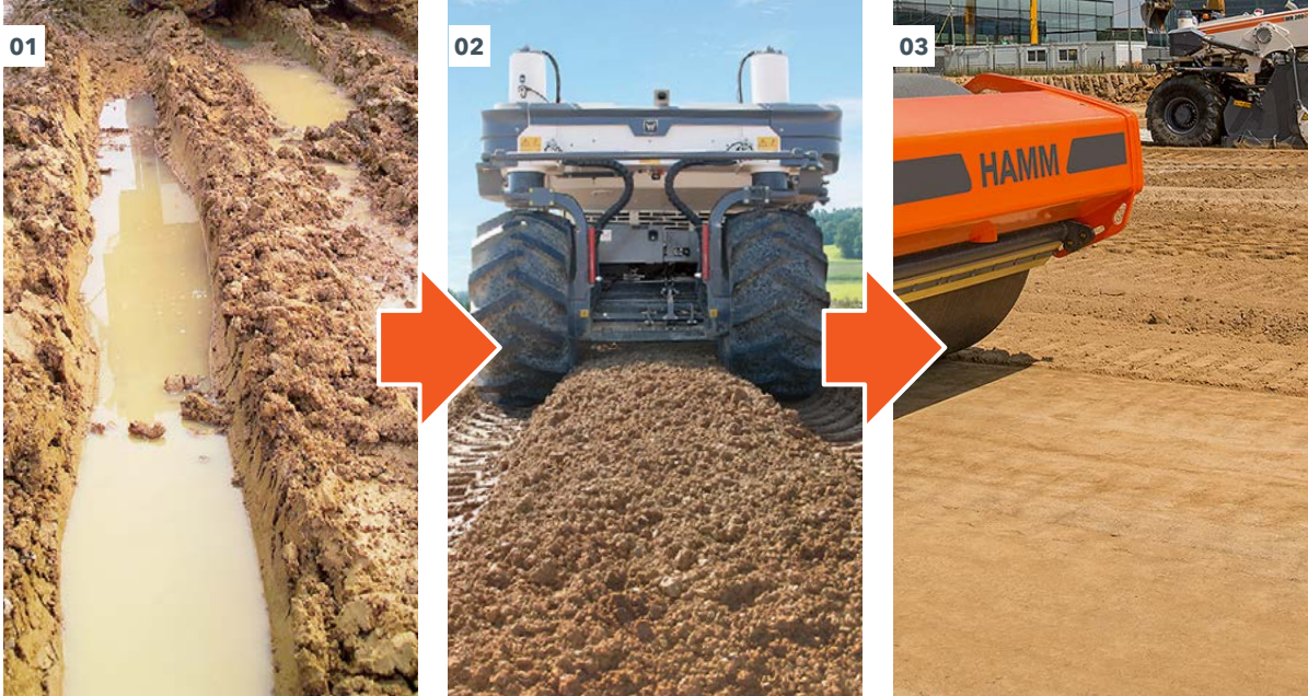
01 - 04 Soil stabilization involves transforming sub-bases with insufficient bearing capacity into soil that is perfect for paving and compaction.
